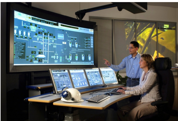
CCTV system protection
